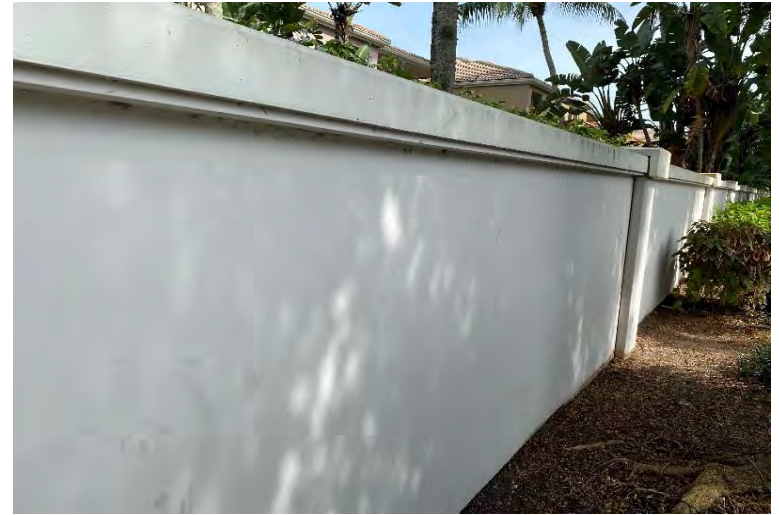
Canal Side Perimeter Wall & Eastside Perimeter Walls
