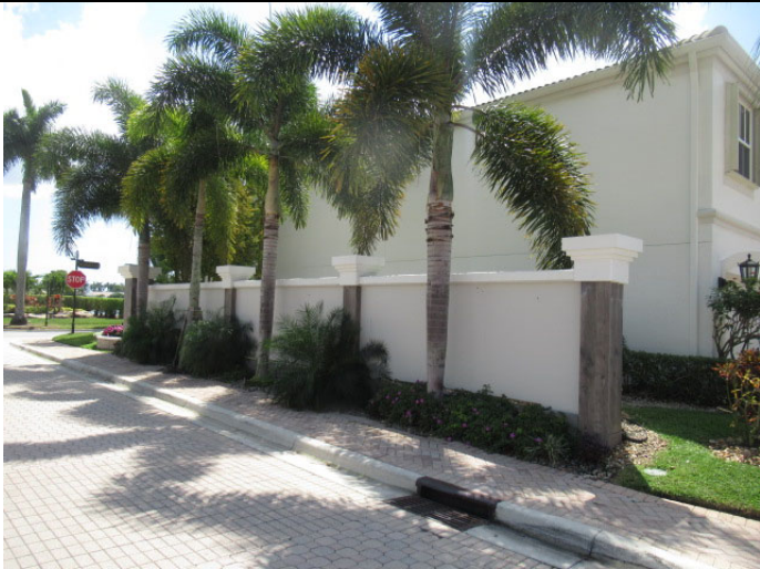
Fencing/Walls and columns
